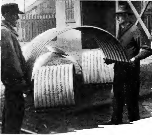
Two men handling a 48-inch diameter "ACME" (Nestable) Corrugated Culvert. Imagine the convenience in handling large culverts in this manner.
